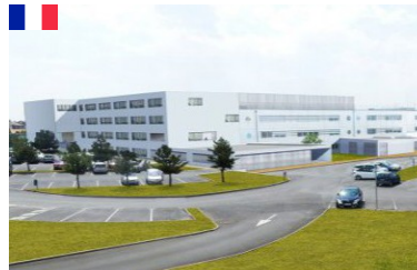
Extending and renovating the Clinique Atlantique (La Rochelle-17) to combine activities with those of Clinique Mail
